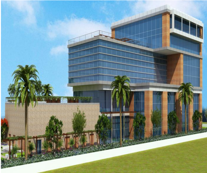
COMMERCIAL PROJECT AT GURGAO
